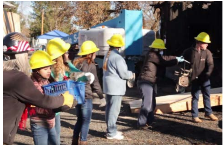
Top: The rebuild and restoration of the 1872 Butte Creek Mill in Eagle Point continues after a devastating fire in December 2015. Above: The week after the fire, the community came out in force to sort through and save anything that survived.
